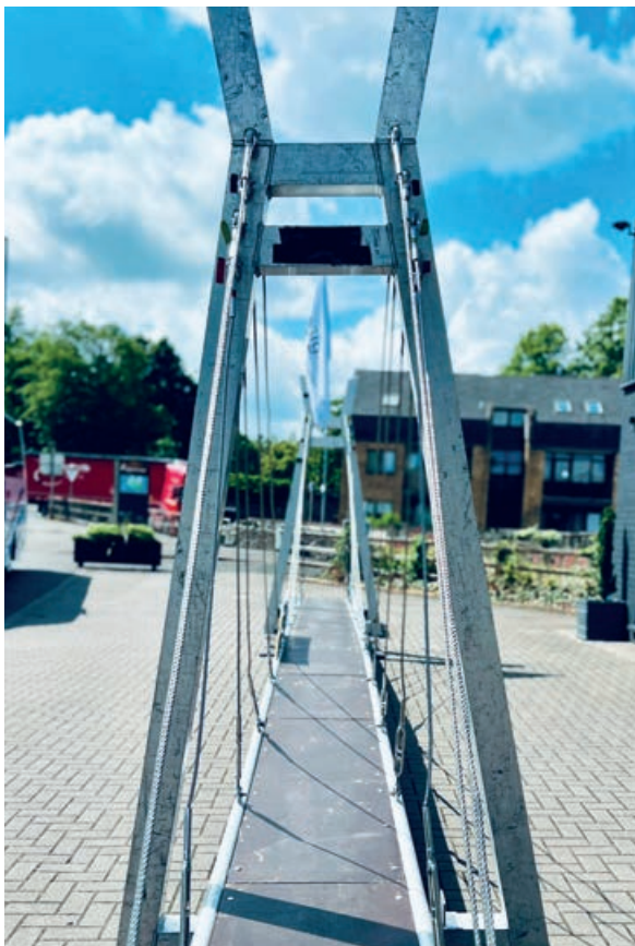
The Big Bridge Project takes its cable-stayed bridge kit to schools for students to build
